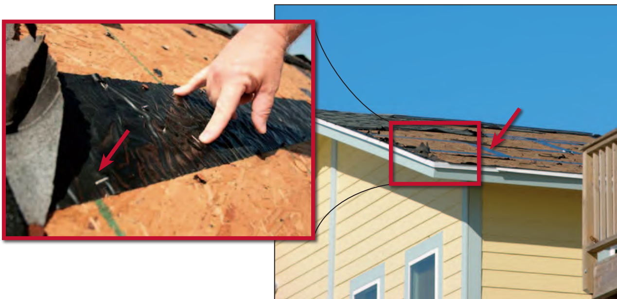
Figure 11-28. House that used enhanced underlayment Option 3 with taped sheathing joints (arrow). The self-adhering modified bitumen tape (inset) was stapled because of bonding problems. Estimated wind speed: 110 mph. Hurricane Ike (Texas, 2008)
